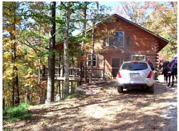
Front Entrance - View of cabin from driveway.
